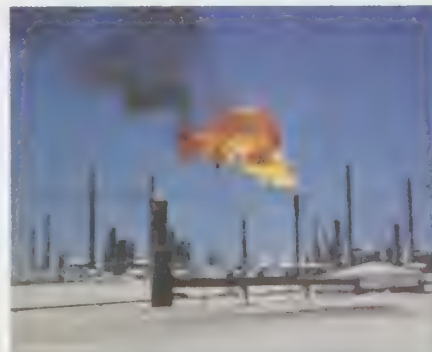
Petroleum refinery at Ras Tanura, Saudi Arabia Herbert A. Banks—Shostal
